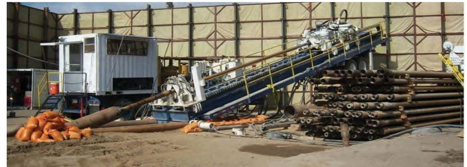
The Lake Oswego Tigard Water Partnership will use horizontal directional drilling (HDD) to construct a new pipeline beneath the Willamette River.
