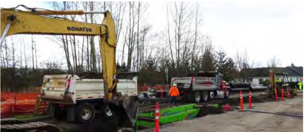
Crews work to install three large water pipelines and a storm drain on Milton Court, which will connect the pump station with the pipelines on Bonita Road.
