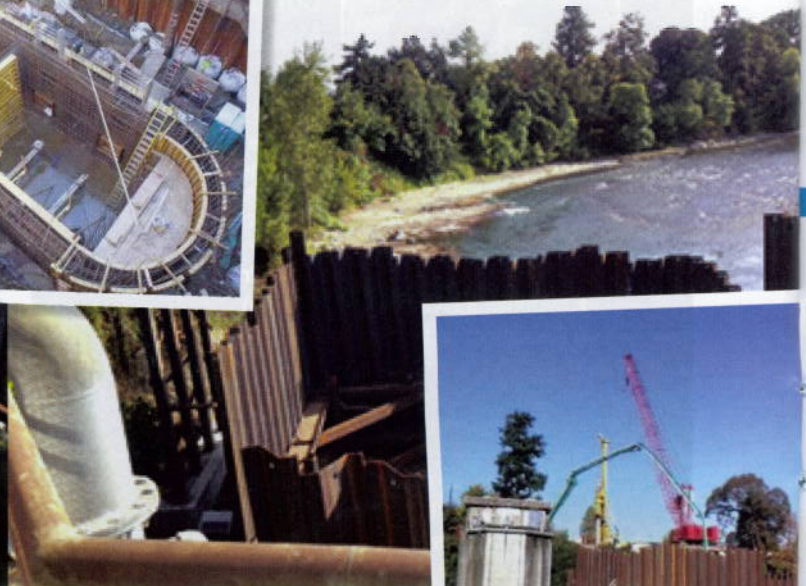
Cofferdam completed (August 21, 2013).
